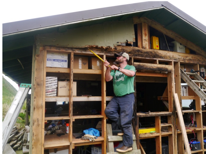
Figure 3. Repairing the Buldir cabin wall.
